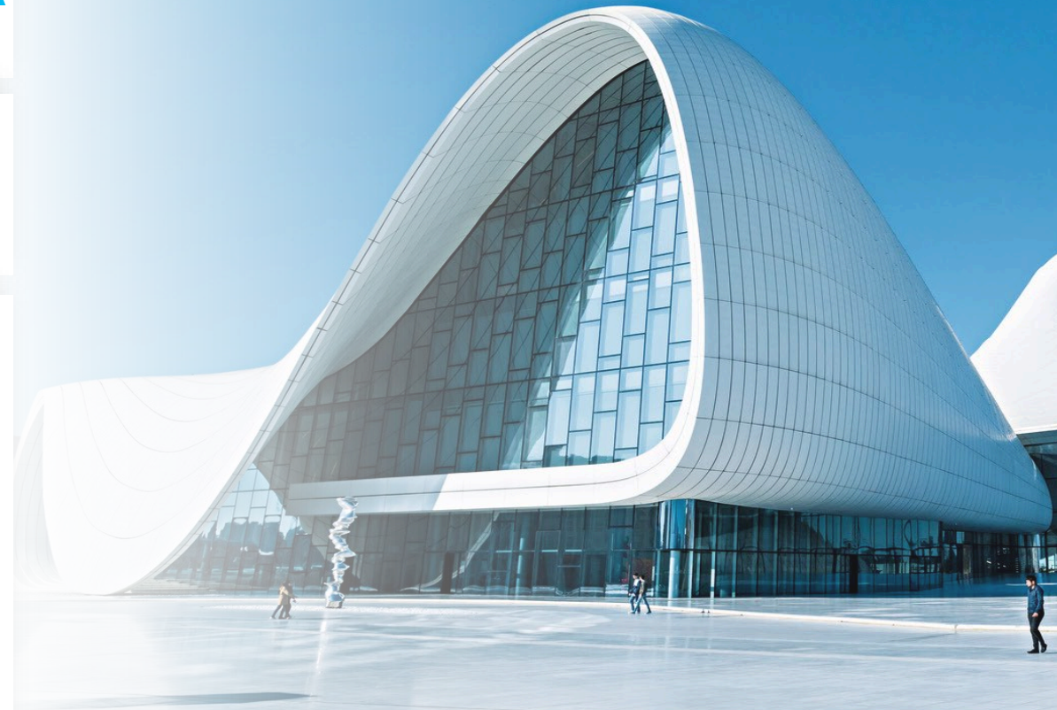
Heydar Aliyev Centre, Baku with Elevate's roofing systems
