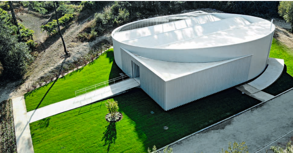
◀ Futuristic Kindergarden, Galicia, Spain – 640 m 2 circular roof was covered with UltraPly TPO thermoplastic roofing membrane
