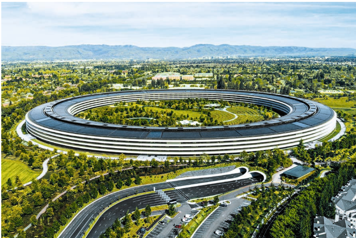
◀ Elevate solar roof at Apple Park, Cupertino, USA
