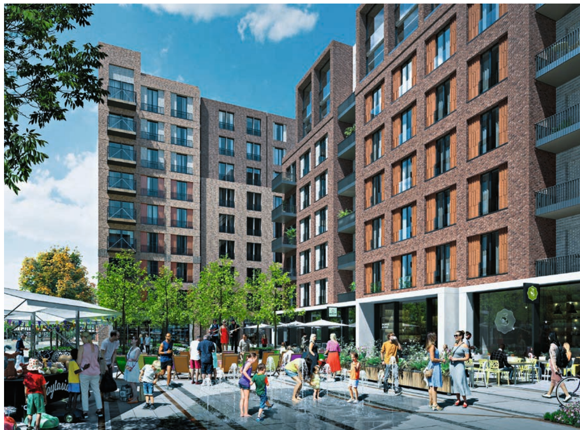
◀ Eight Gardens, London that has ECOPact green concrete inside with 64 percent lower CO 2
