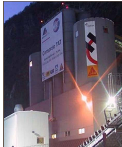
Partner for the tunnel construction and not merely CEM supplier
