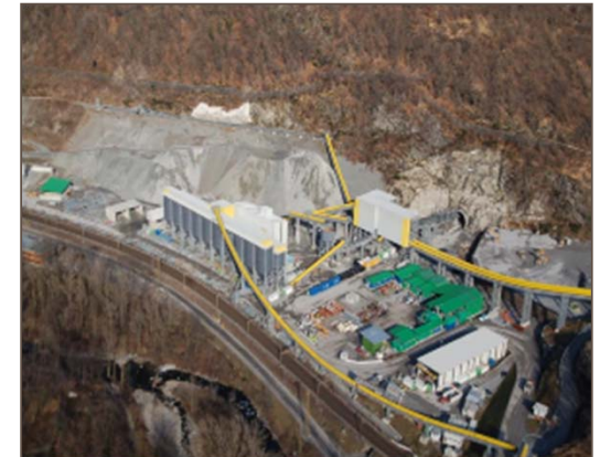
Excavation material handling
