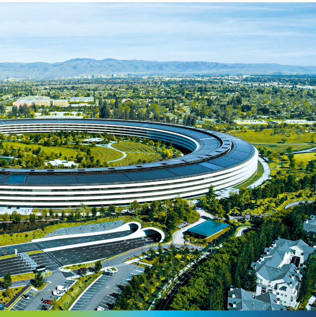
Firestone solar roof at Apple Park, Cupertino, USA
